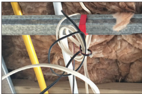
Typical cable installation
